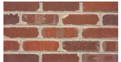
Standard 3/8" Mortar Joint
