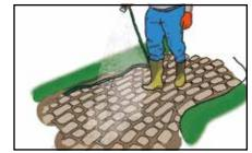
6. **Blow off** any excess water remaining on the paver pores and crevices.
